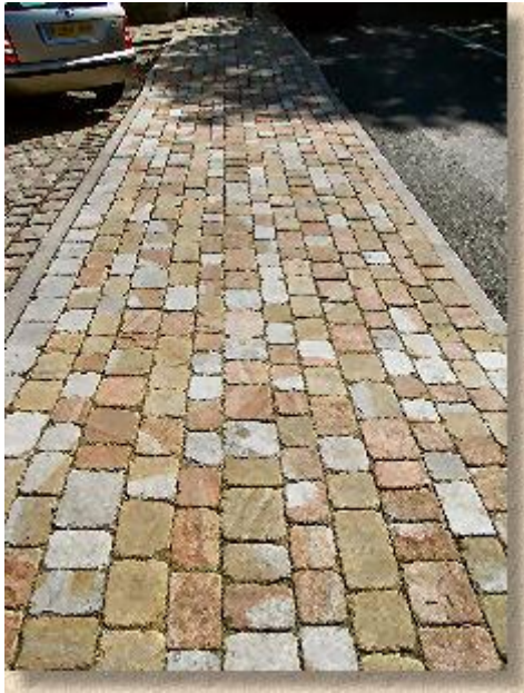
Flexible sett paving laid to a vehicle crossing
