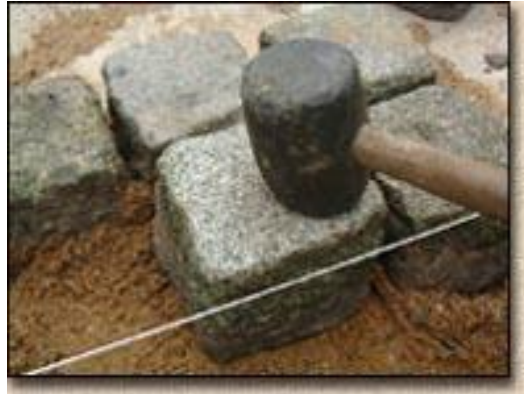
Place Sett and tap down to level
