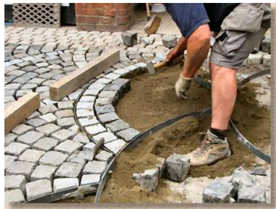
Standard scale fans are often laid using a template frame
