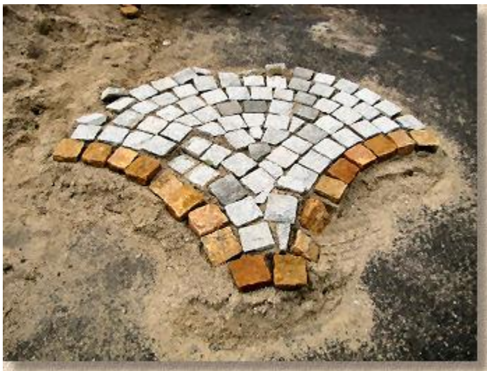
Fans are usually mocked-up to check scale, contrast and joint width
