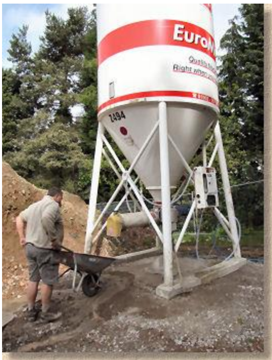
Mortar silo used on larger projects to dispense a consistent bedding material
