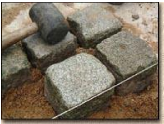
Check level with line guide
