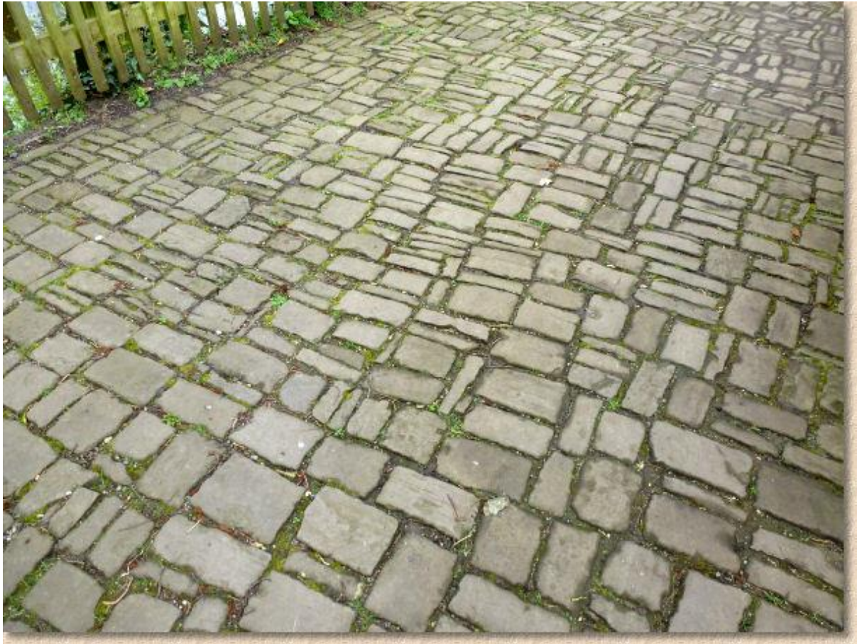
Random laid setts, although some of the blocks of this laminar stone have split in-situ, enhancing the random look
