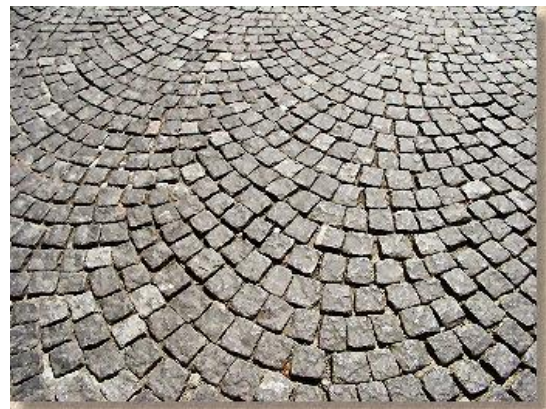
Cubes laid in bogen pattern
